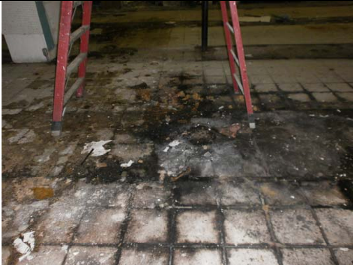
First Floor Mold Growth
